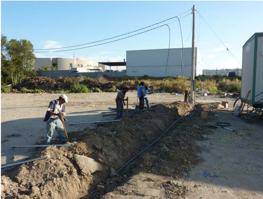
Workers installing metal posts for fence, next to electrical cables buried underground.
